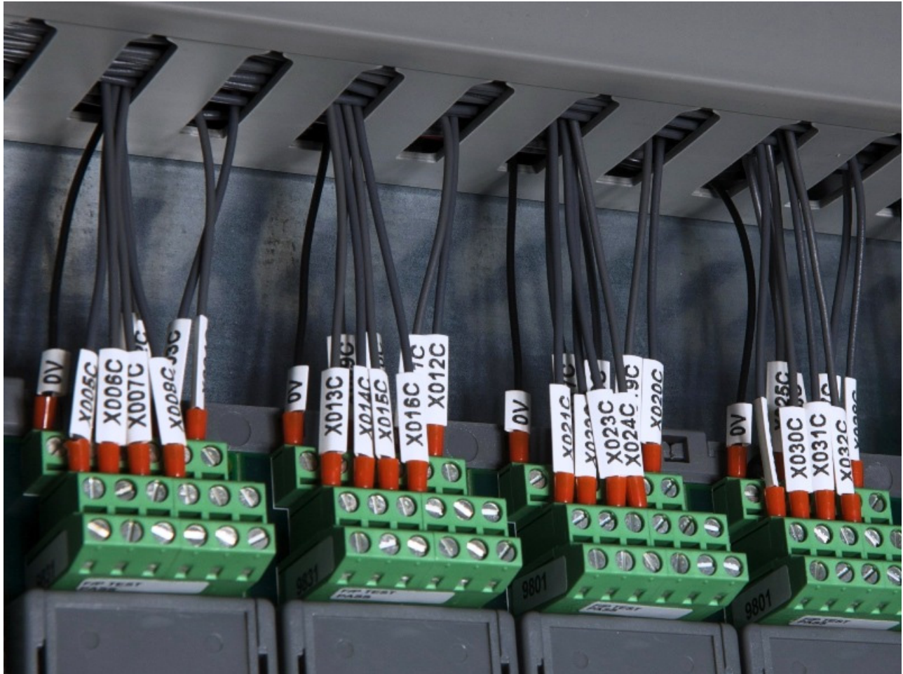
Figure 5 - Field Wiring Connections
