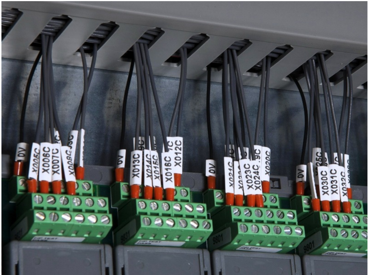
Figure 13 - Field Wiring Connections
